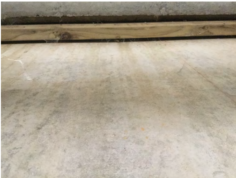
Gap between deck panel and ballast wall on right bank filled with treated timber
