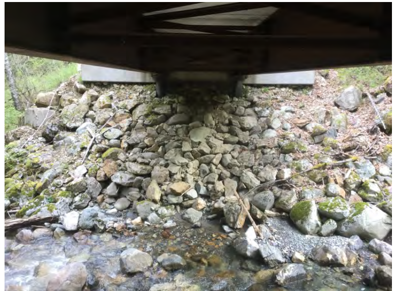
Right Bank Abutment when facing downstream
