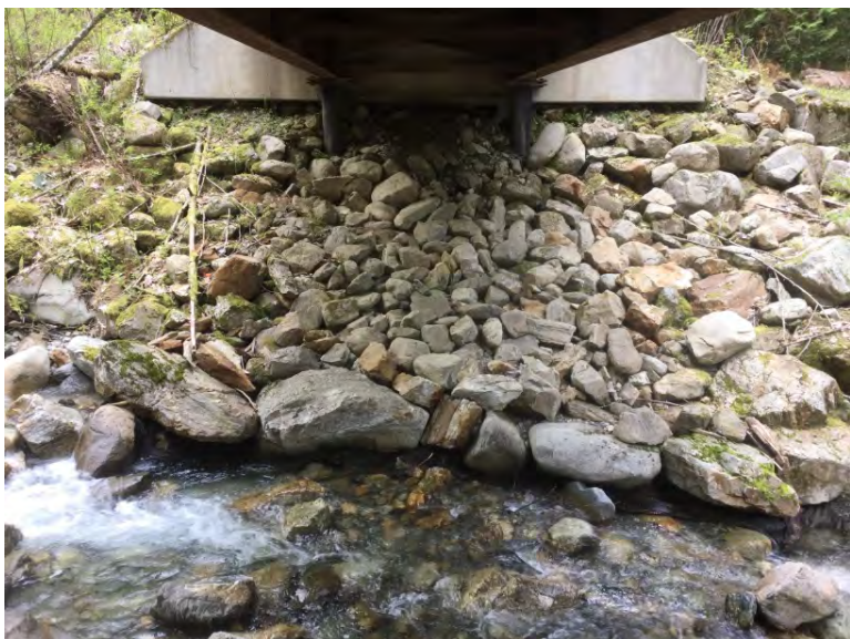
Left Bank Abutment when facing downstream
