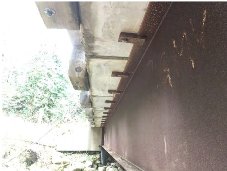
Deck clips in place and functional
