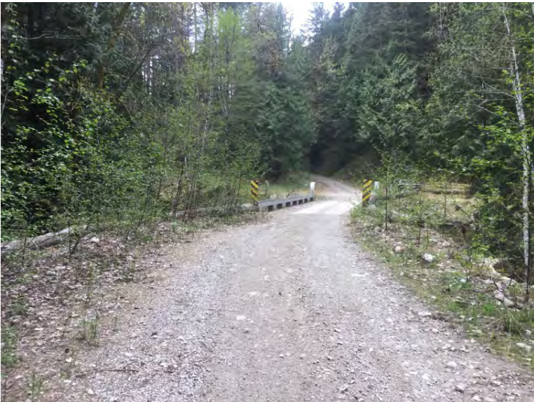
Approach from Right Bank when facing downstream
